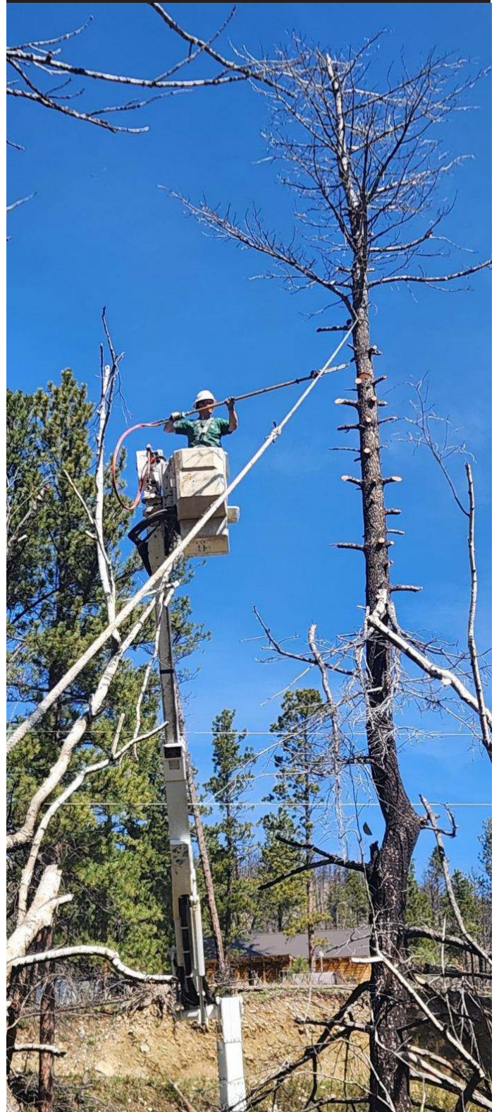
Big Flat Electric Lineman Nathan Veit works tree and line maintenance in the Landusky area. | PHOTO BY LEIF SORENSEN
