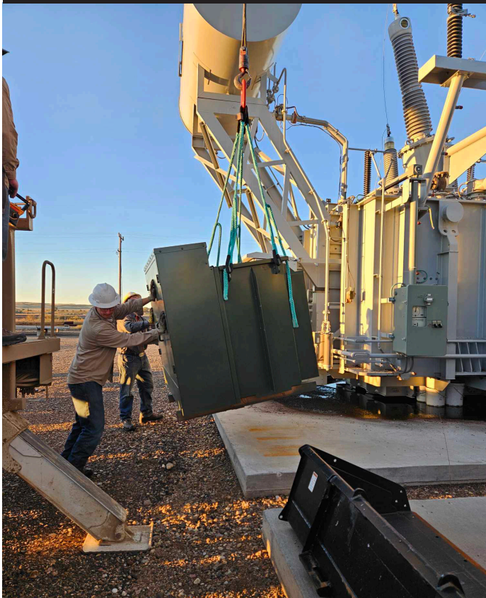
ABOVE: BFEC linemen unloading a 225 KVa 3-phase pad transformer.
