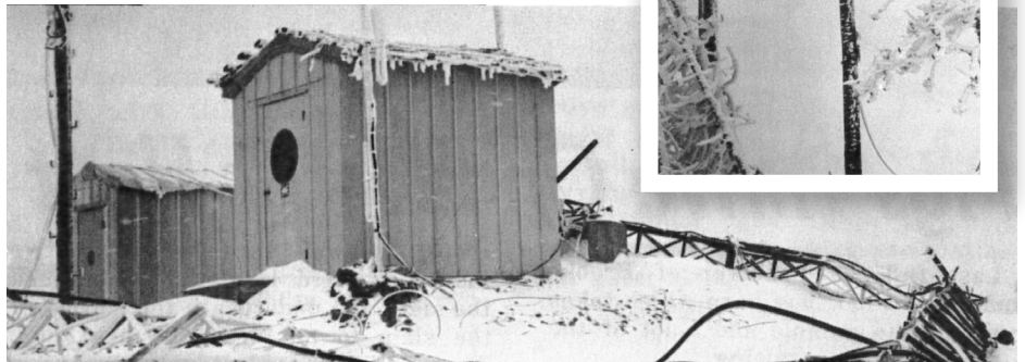
The twisted wreckage of the 160 ft Boarder Patrol radio tower and equipment building. Little damage was suffered by the buildings as the tower collapsed in a spiral around them.
